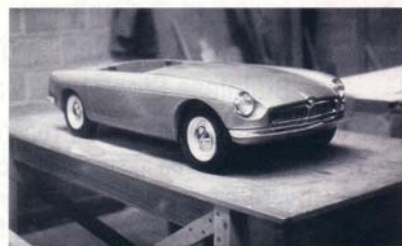
Original EX 214 – MGB Quarter Scale model taken in development – first view of MGB shape. Photo Don Hayter.
